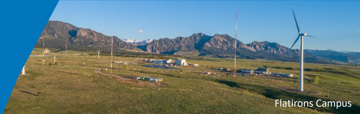
Energy Systems Integration Facility (ESIF)
