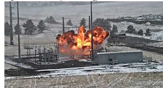
Substation device failure forced stand-alone microgrid operation at NREL Flatirons Campus
