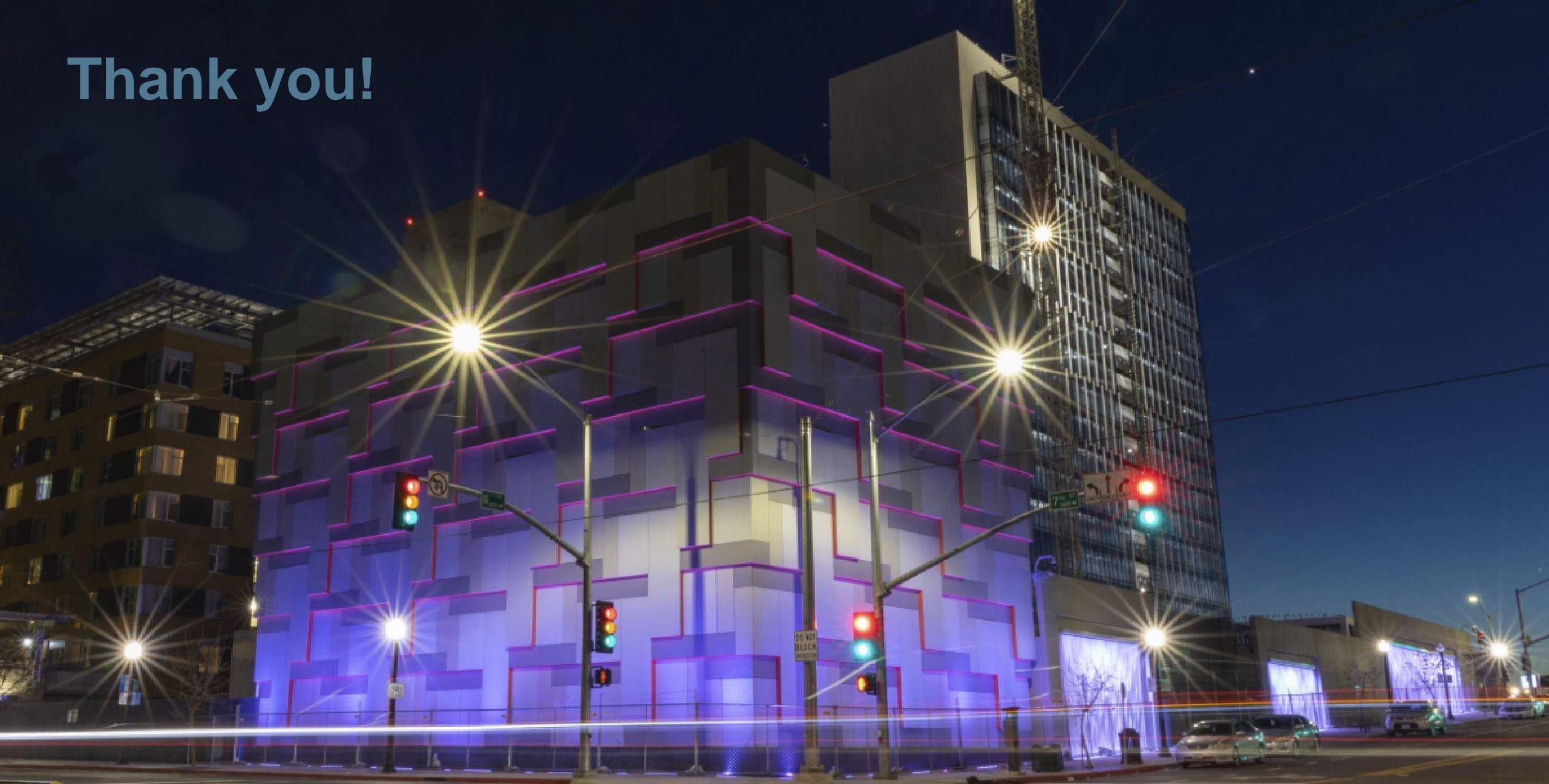
18 Bulk Substation "Station G"
