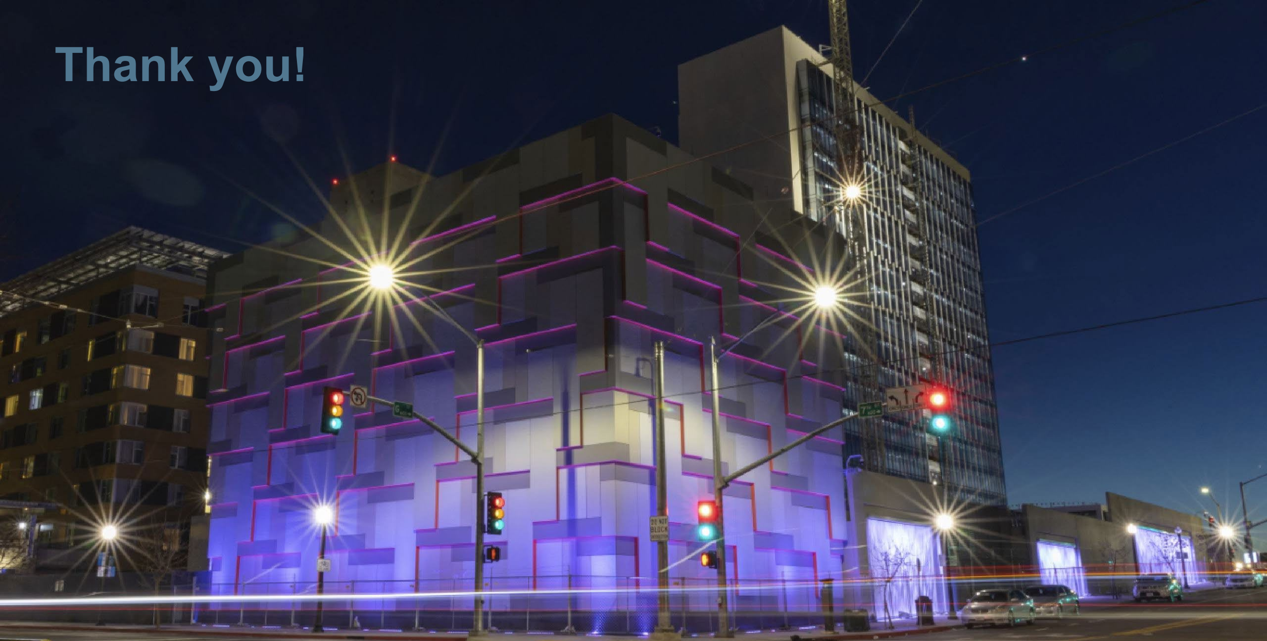
12 New Bulk Substation "Station G"
