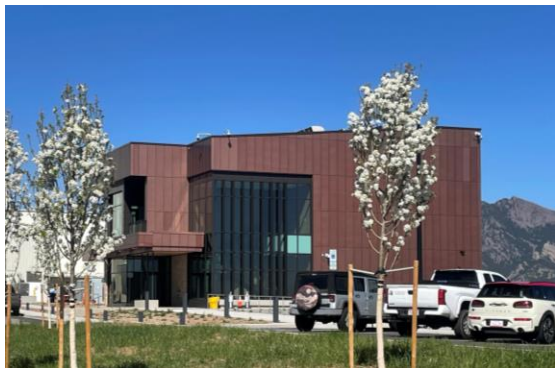
Control Center Facility – Robb Wallen / NLR
