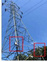
No outage required for LineVision installation (devices install near the base of the transmission tower)
