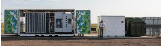
Inverter can operate in both GFM and GFL modes
