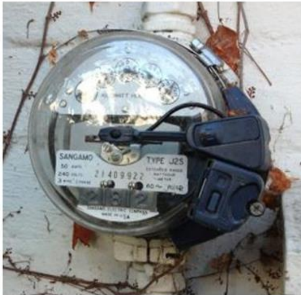
Utility approved Blueline device attached to utility meter.
