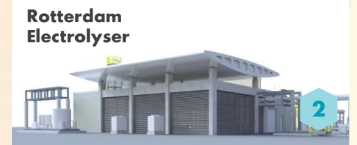
Maasvlakte 200 MW on stream 2023
