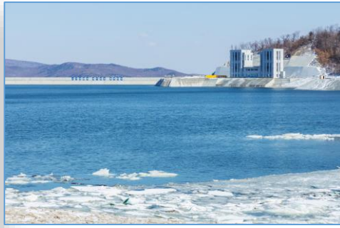
Mudanjiang pumped plant
