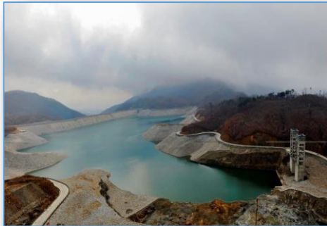
Pushihe pumped plant
