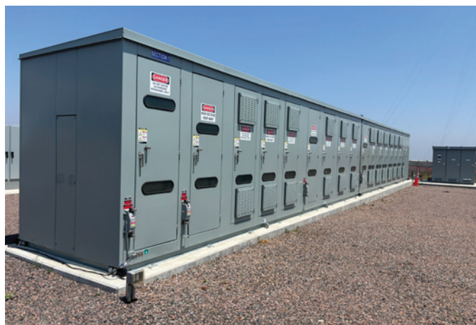
FIGURE 6 Medium-Voltage Impedance Network Capable of Emulating Weak-Grid Conditions
